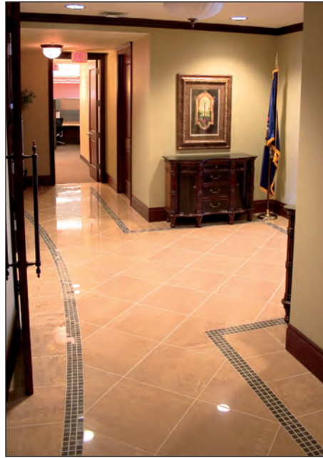
Polished porcelain tile, with a dark gray mosaic tile inlay, carries through to an inner foyer and hallway leading in one direction to the executive offices, and in the other to the sales offices.
